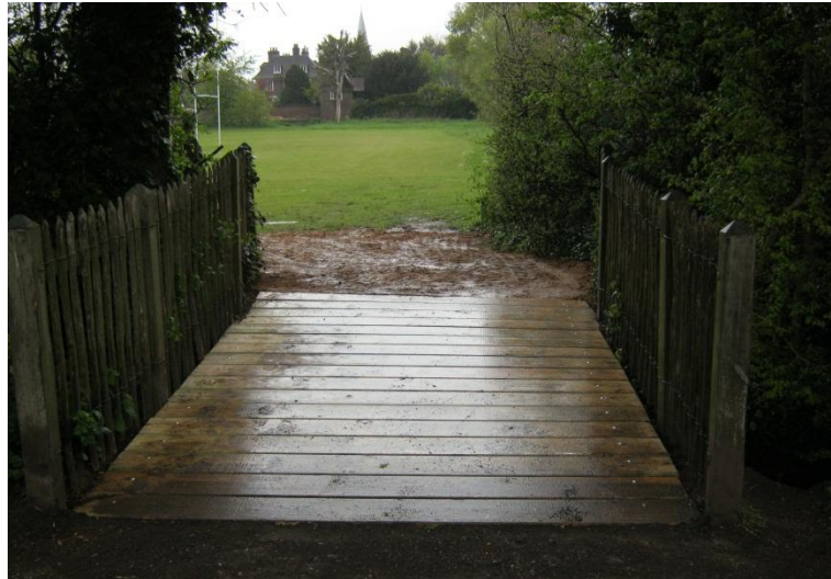
Figure 2: Re-built Hampstead Heath Extension Bridge.
